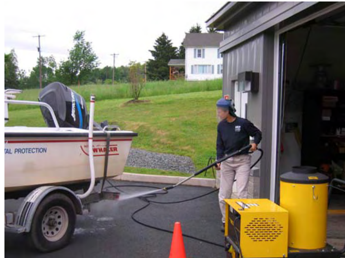
Figure 5.7 Steam cleaning a boat to prevent transport of zebra mussels.
