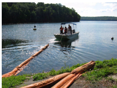
Figure 3.3 Wave stabilization boom installation.
